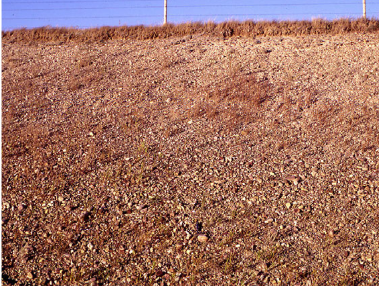
Figure 14.12. Close up of the gravel cap in Figure 14.11. Most of the rocks are low-grade quartzite rocks from east of the continental divide.
