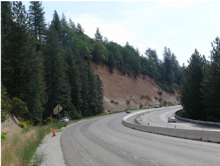
Figure 25.6. Gravel layer in the western Sierras along I-80 east of Sacramento, California.
